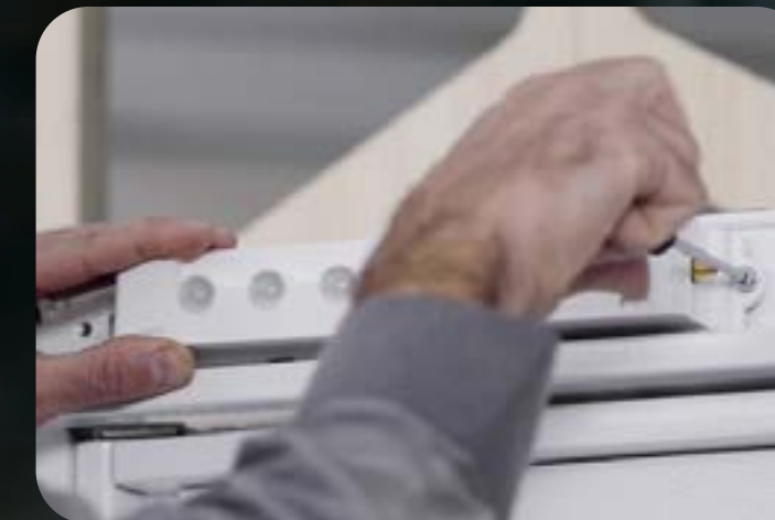
Step 1: Install the wireless server on top of the frame with two screws
